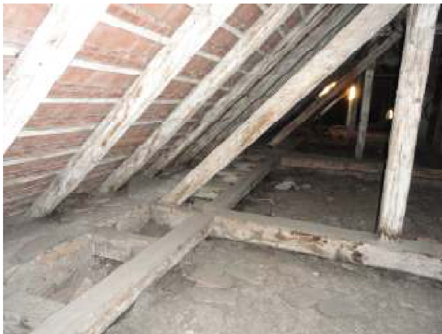
DETALIU SARPANTA - GRINZI COARDA, ARBALETRIER, POP, CAPRIORI, LONGERON
