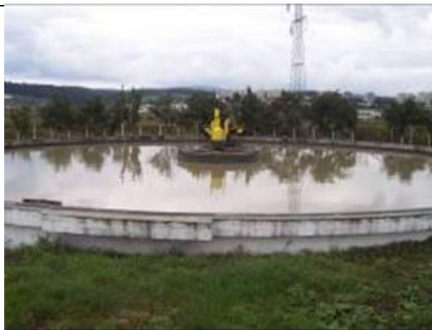
Figura 71 – Decantor primar radial
