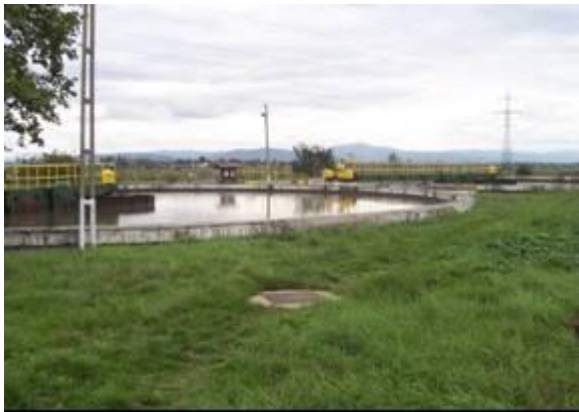
Figura 73 – Decantor secundar radial
